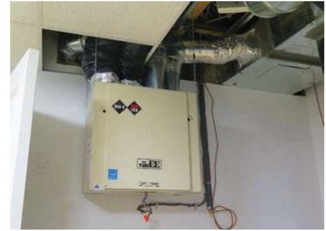
ERVs provide ventilation, heat recovery and humidity control.
