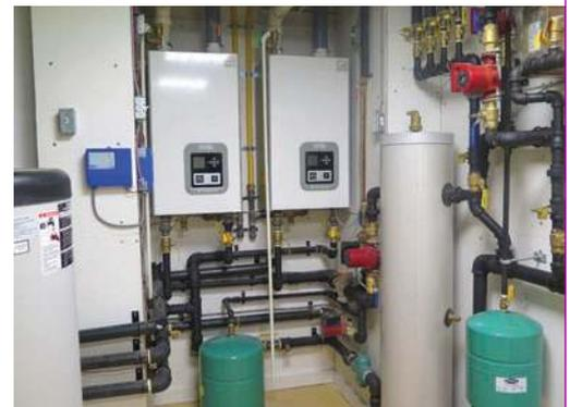
Two boilers and four air handlers make up the heart of the HVAC system.
